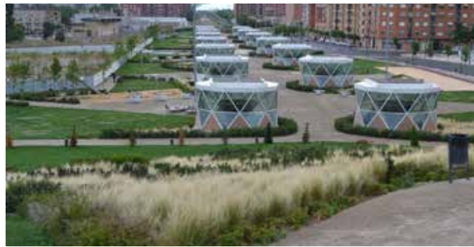
AVE RAILSTATION - SPAIN
