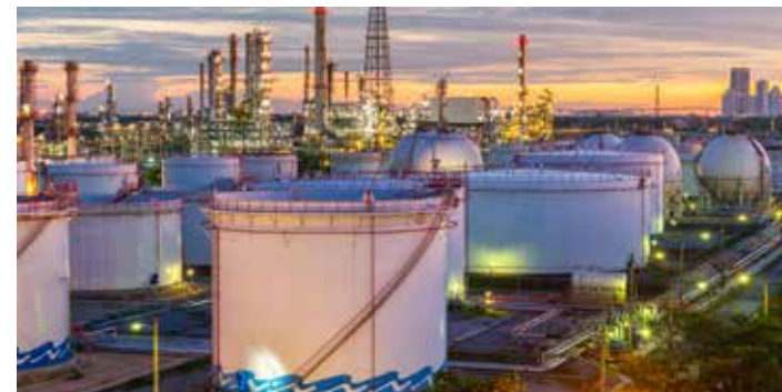
OIL&GAS FACILITIES - QATAR
